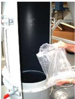
Figure 6 Applying cleaning pellets into extract duct
