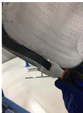
Figure 12 Removing old seal and preparing the surface
